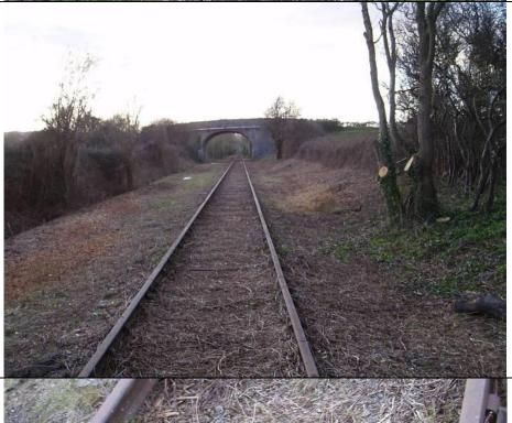
The third of the heavily engineered GWR bridges that remain over the line. Note the permanent way width: wide enough for two broad gauge tracks.
