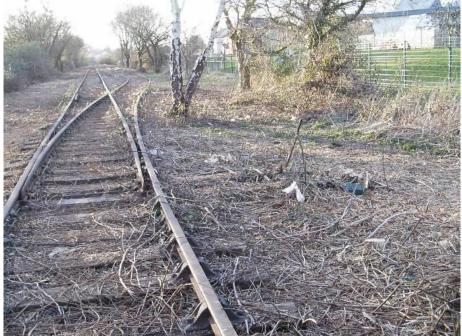
The single track becomes doubled to form a passing loop. The points operating lever is to the right of the line, beyond a piece of rubbish.
