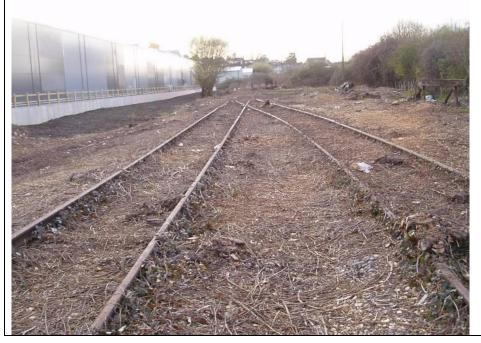
The twin tracks converge at points near the end of the line. These points and the previous points provided a "run around" track for a locomotive.
